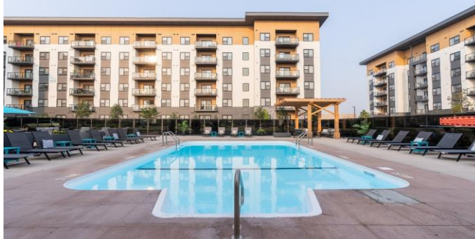
Vibe Apartments 90 Arbour Lake Hill NW, Calgary
